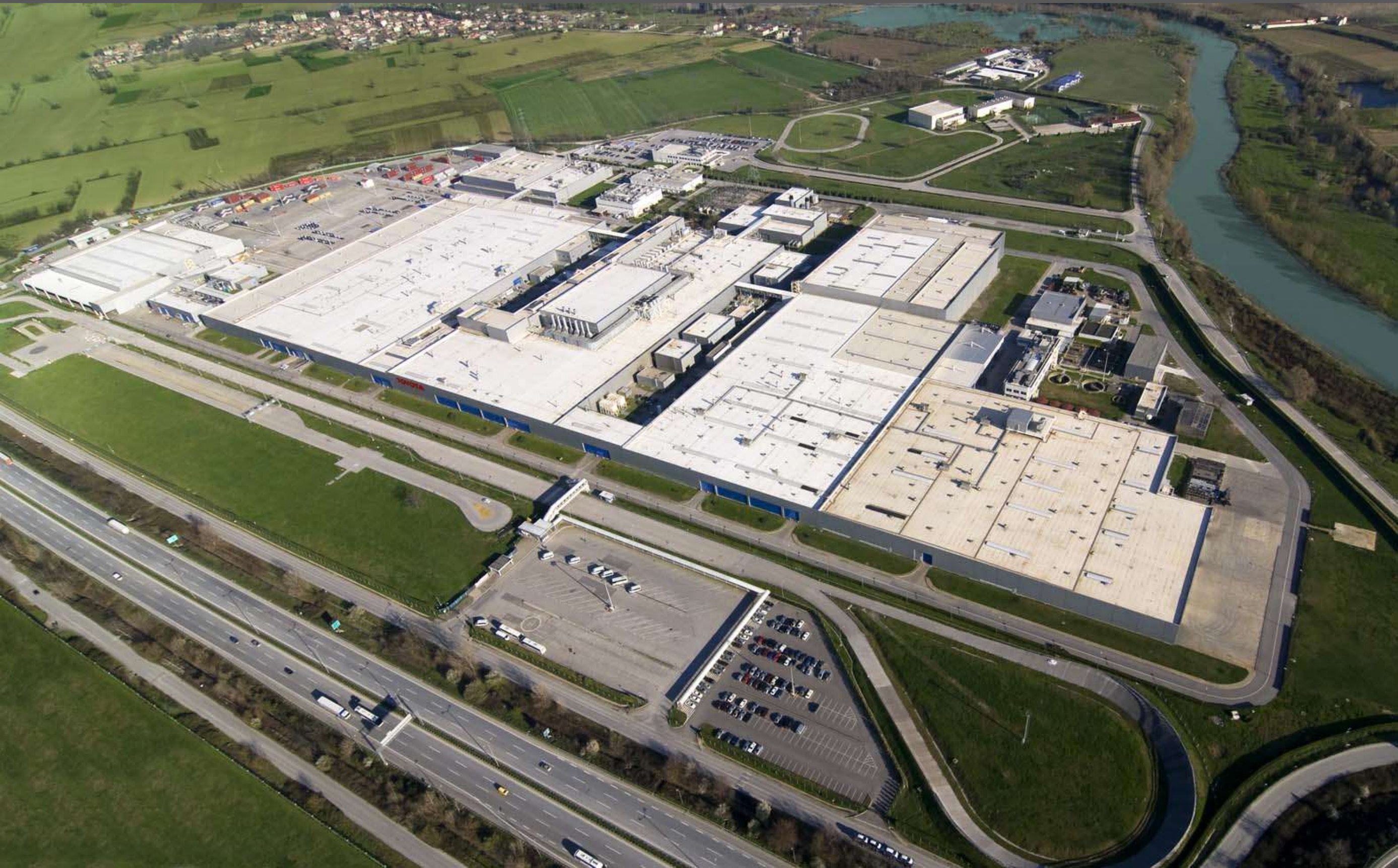
TOYOTA CAR FACTORY- ADAPAZARI-TURKEY AUTOMATIC WELDING MACHINES ERECTION & HVAC SYSTEMS
