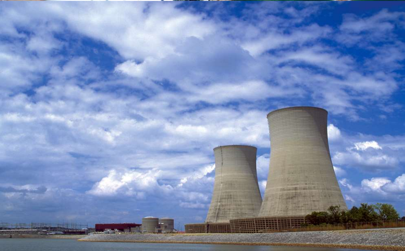
COOLING TOWER PROJECT BAKU / AZERBAIJAN
