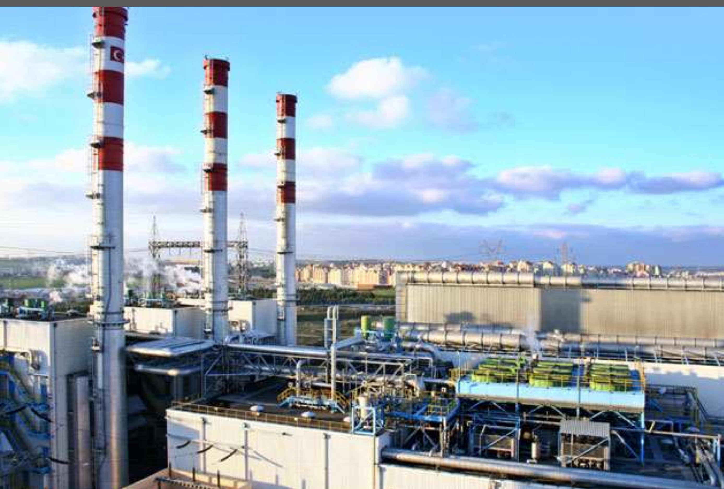
ISTANBUL ESENYURT CCPP POWER PLANT 180 MW
