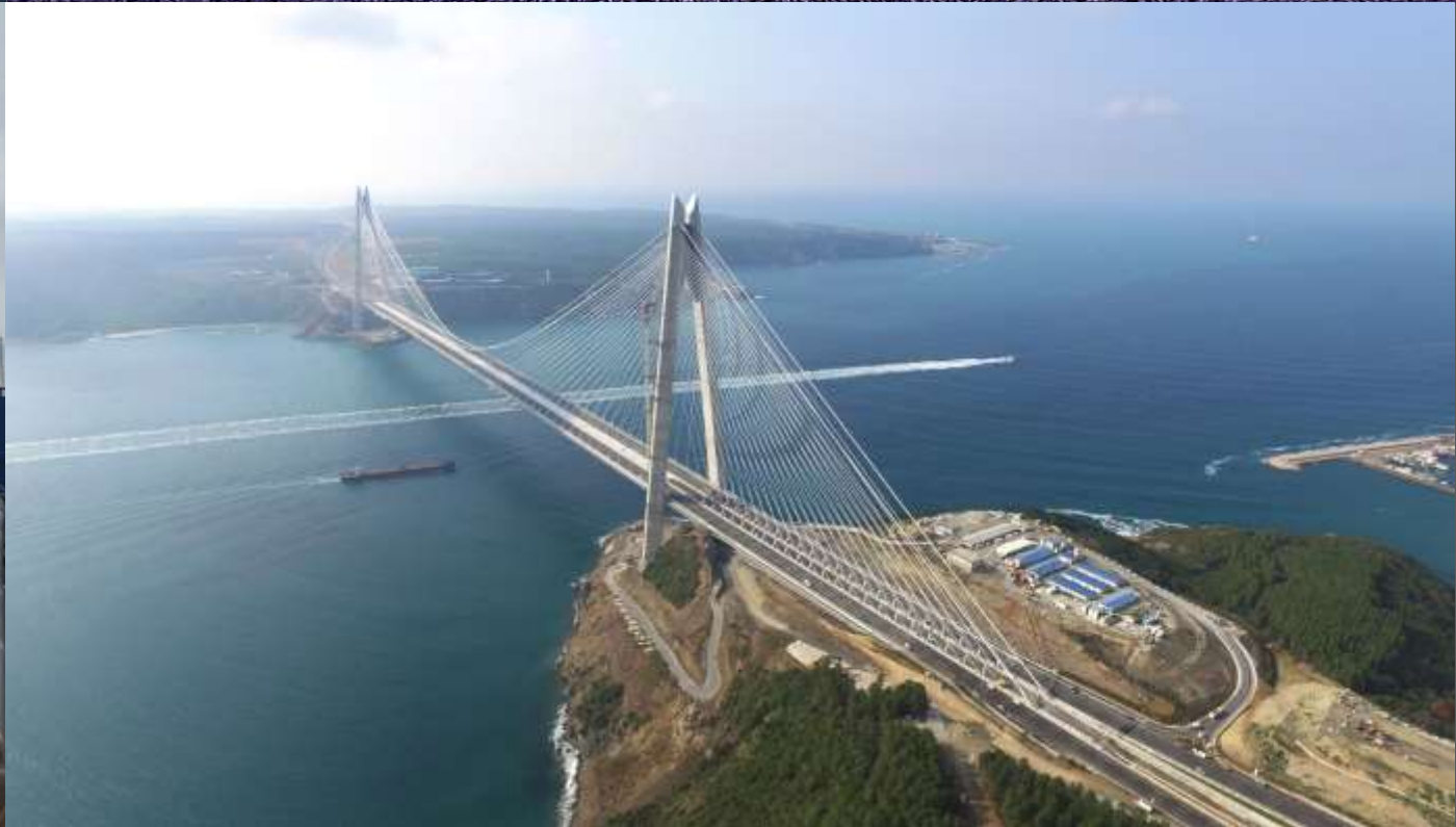
YAVUZ SULTAN SELIM BRIDGE ISTANBUL / TURKEY
