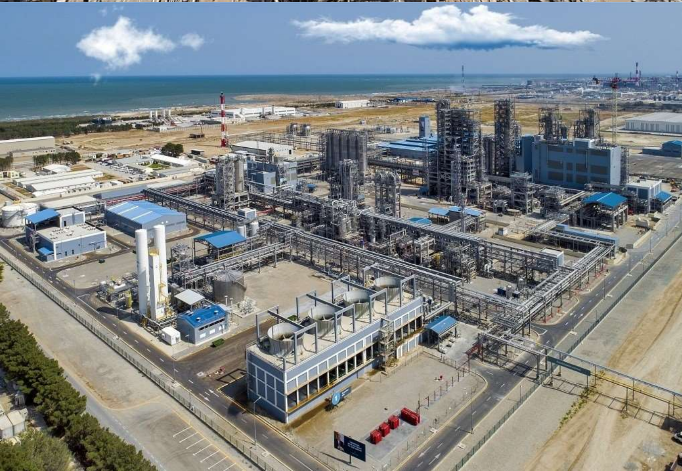
SOCAR HDPE PLANT SUMGAYIT / AZERBAIJAN
