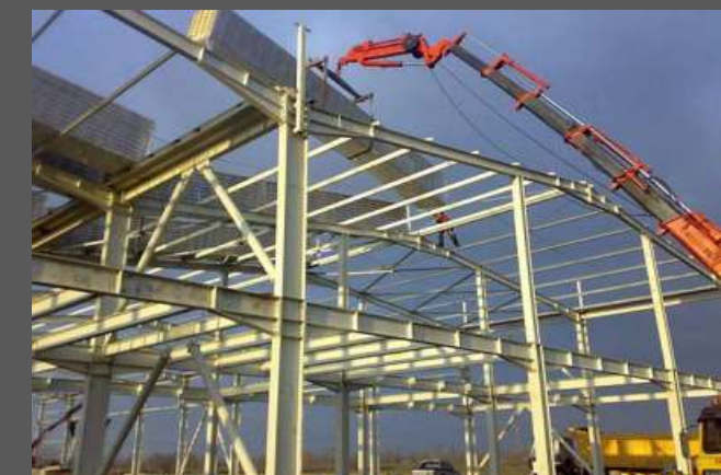
STEEL BUILDINGS CONSTRUCTION
