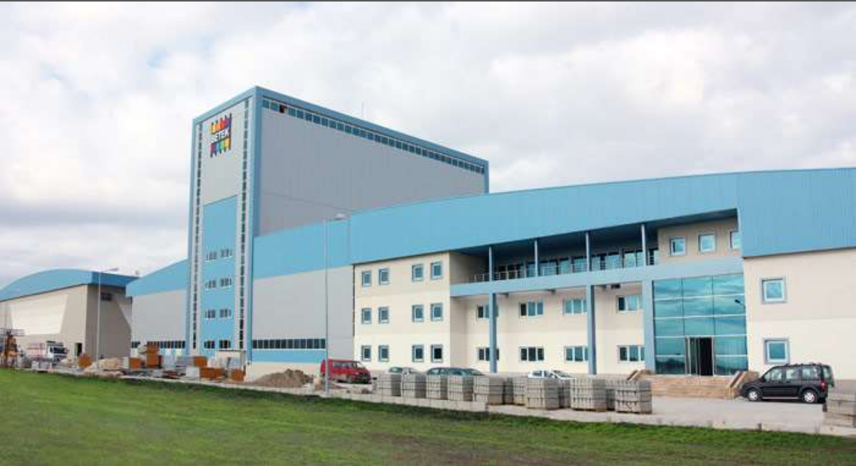
BETEK BOYA PAINT FACTORY -IZMIT-GEBZE
