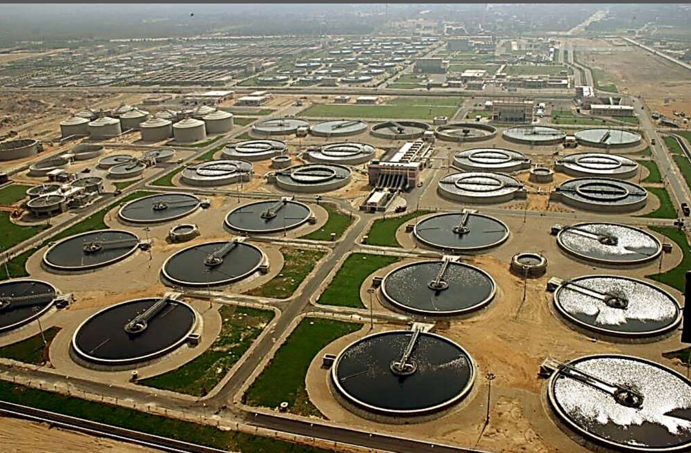
ABU RAWASH WASTE-WATER TREATMENT PLANT CAIRO/ EGYPT
