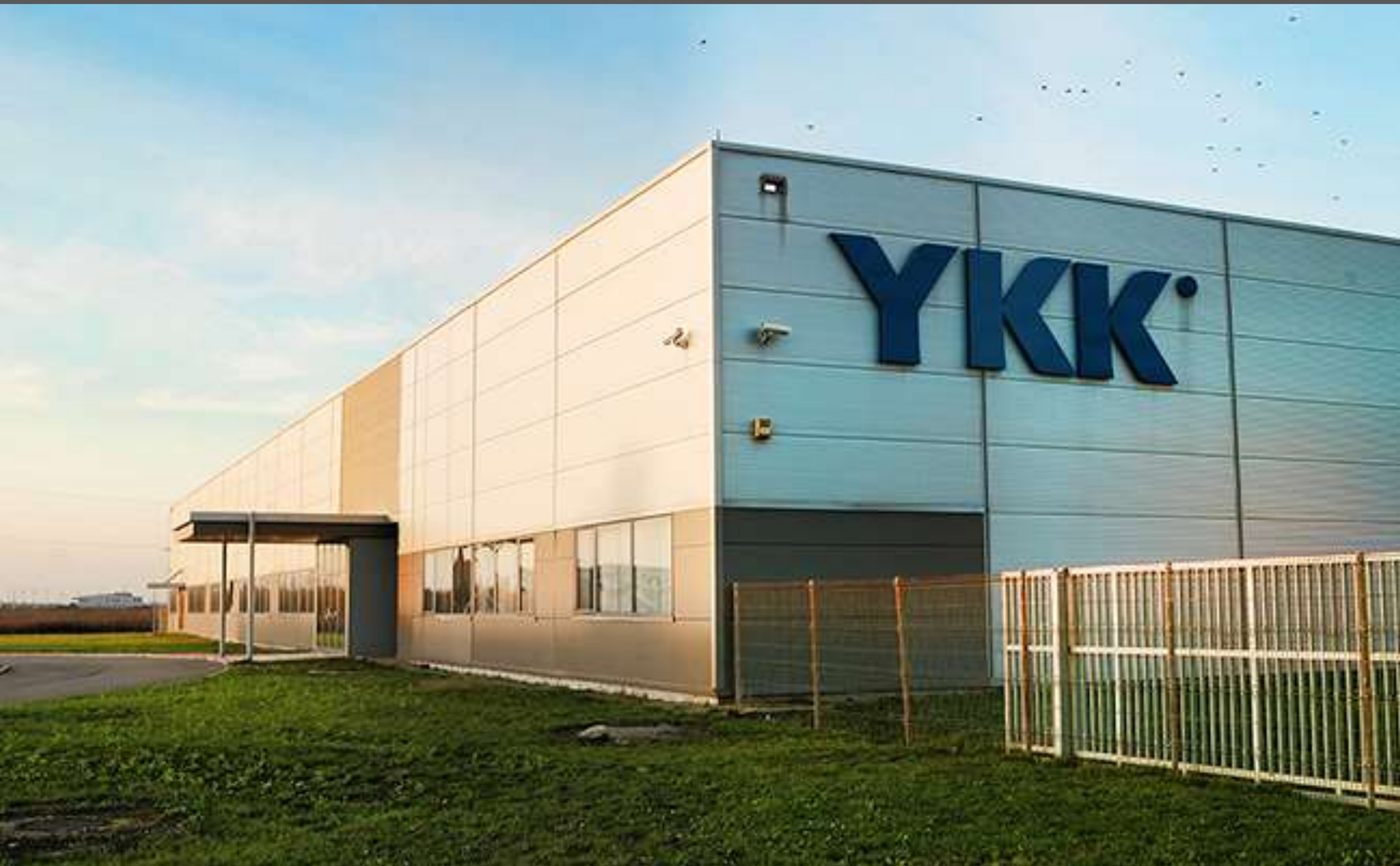
YKK ZIP FACTORY CORLU-TURKEY MECHANICAL WORKS
