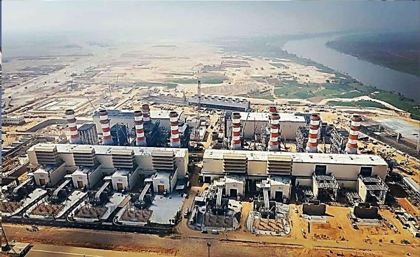
ASSUIT COMBINED CYCLE POWER PLANT / EGYPT
