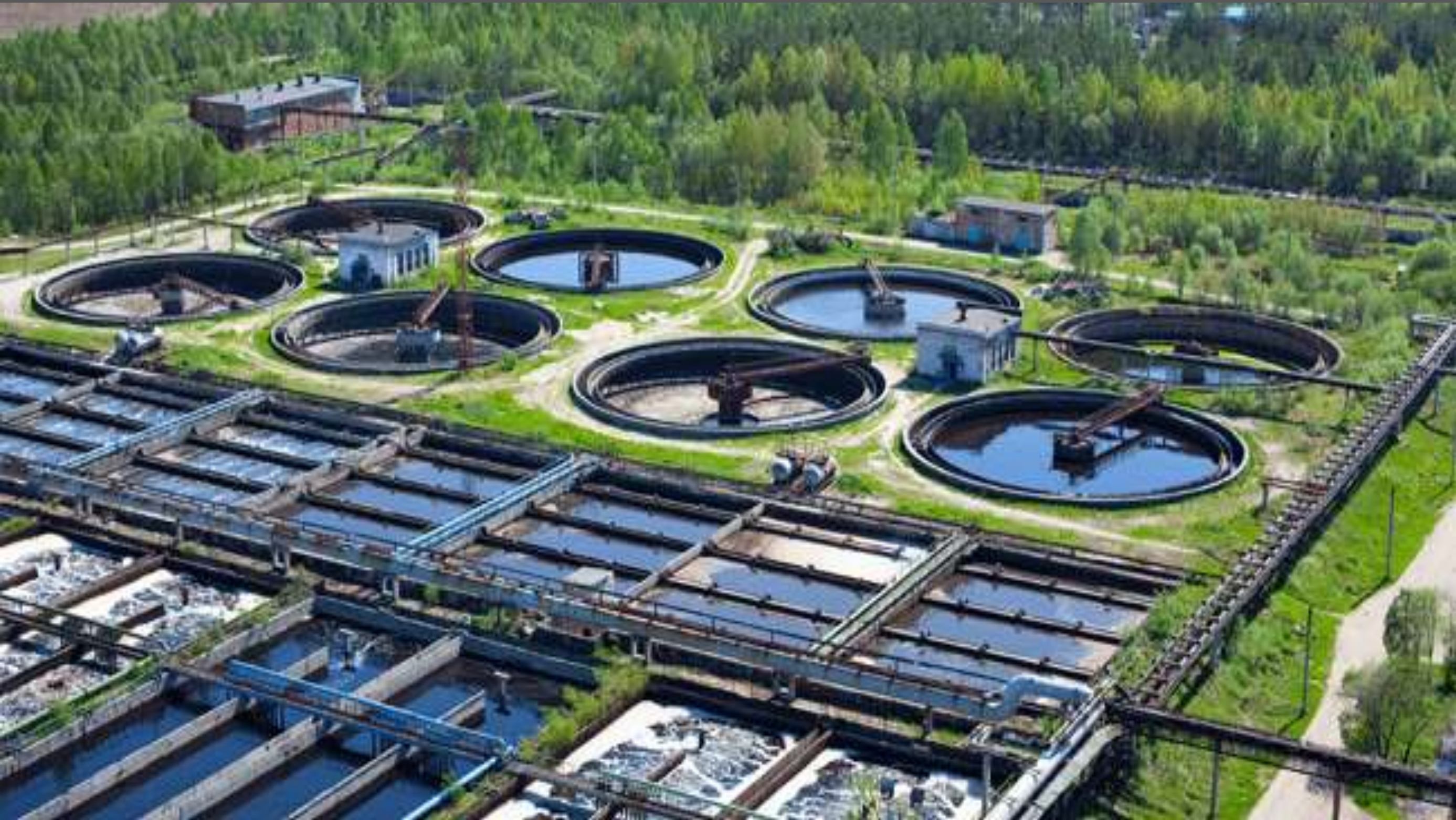
ARAD CITY -ROMANIA WASTE WATER TREATMENT PLANT
