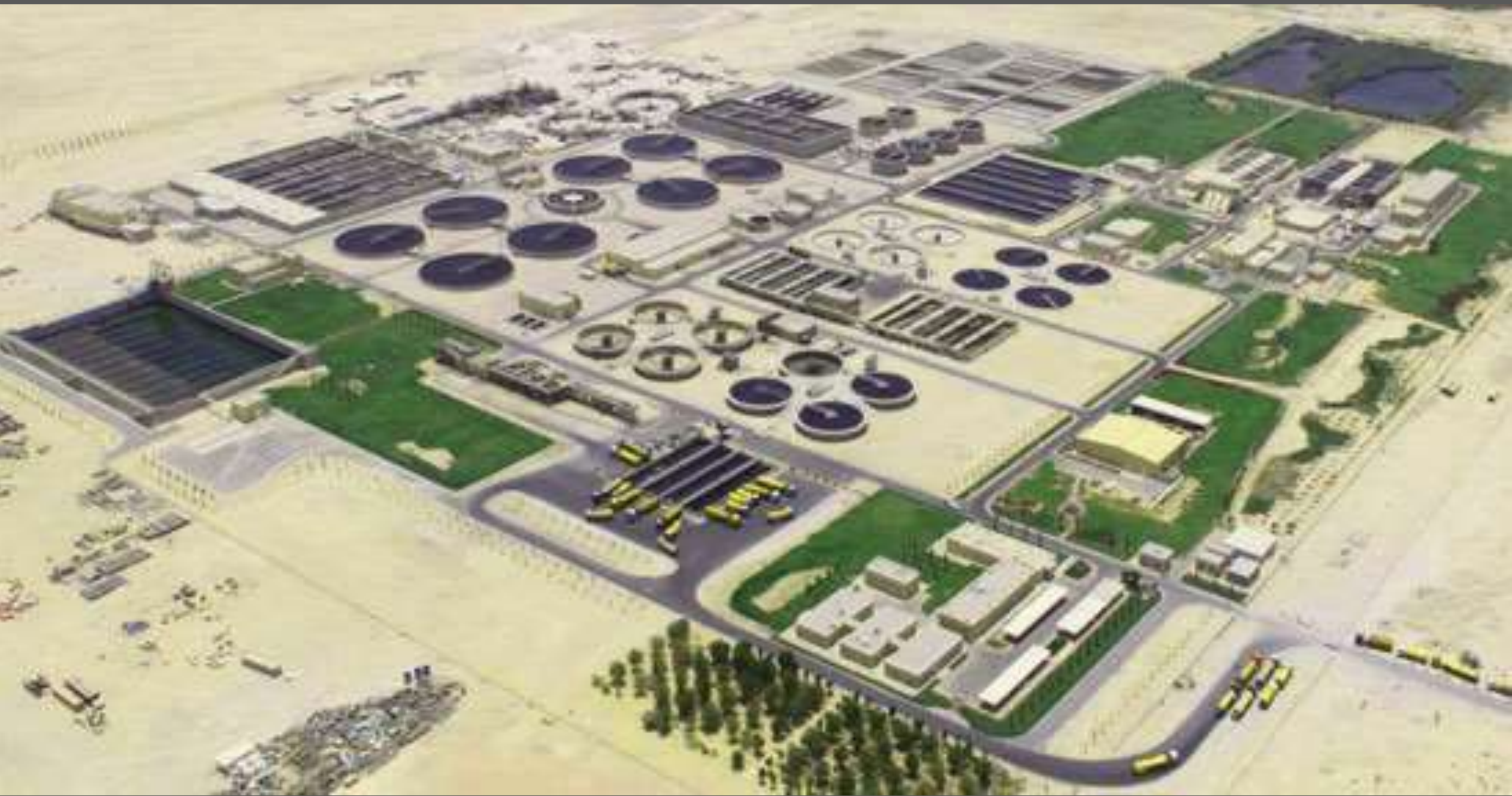
DOHA NORTH SEWAGE TREATMENT PLANT
