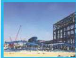
Brullus Power Plant 4800 MW PCESCO / EGYPT
