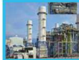
New Capital Power Plant 4800 MW PCESCO / EGYPT
