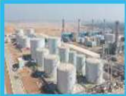
Assiut Add-On Power Plant 500 MW PCESCO / EGYPT
