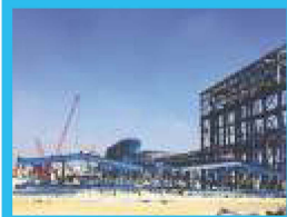
Brullus Power Plant 4800 MW PCESCO / EGYPT
