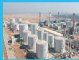
Assiut Add-On Power Plant 500 MW PCESCO / EGYPT
