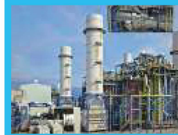
New Capital Power Plant 4800 MW PCESCO / EGYPT
