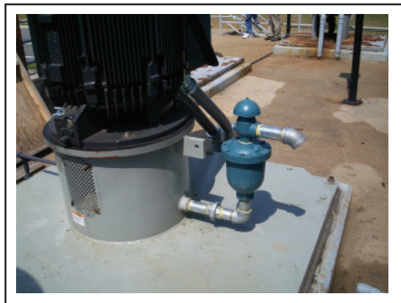
Air/Vacuum Valve with Dual Port Throttling Device
