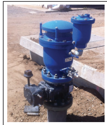
Dual Body Combination Air Valve
